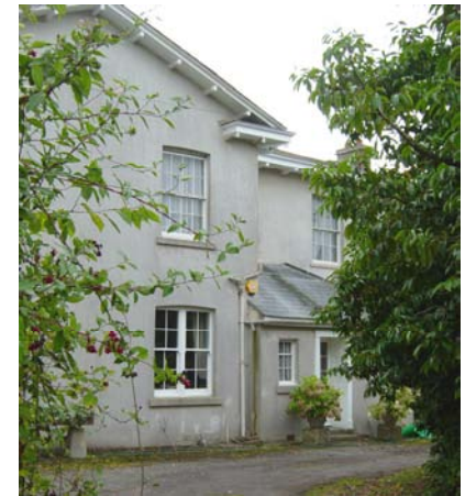
Fig 42. The Old Cottage with sash windows
